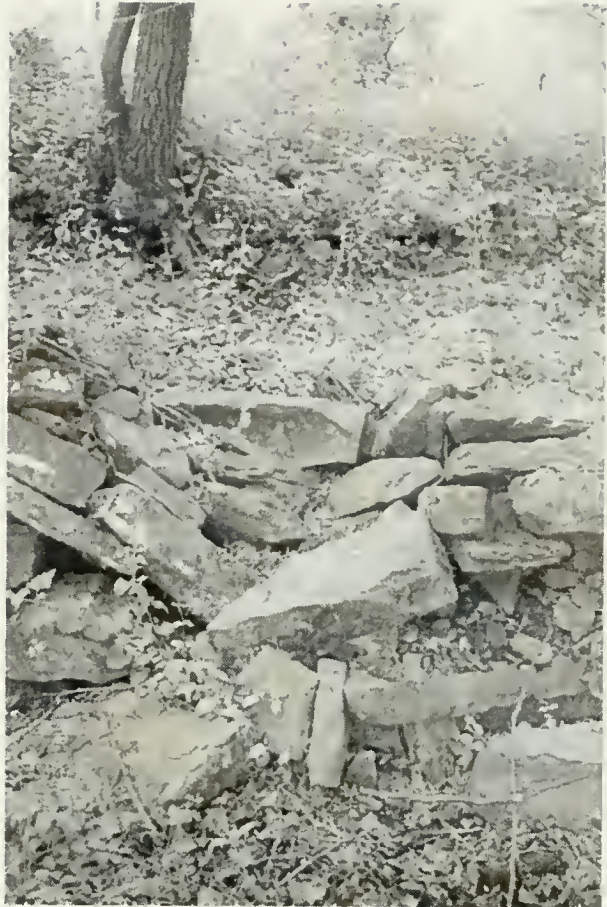
Figure 47 Stonework of the Dam, 2001
